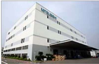
Air Conditioning and Refrigeration Systems Works
